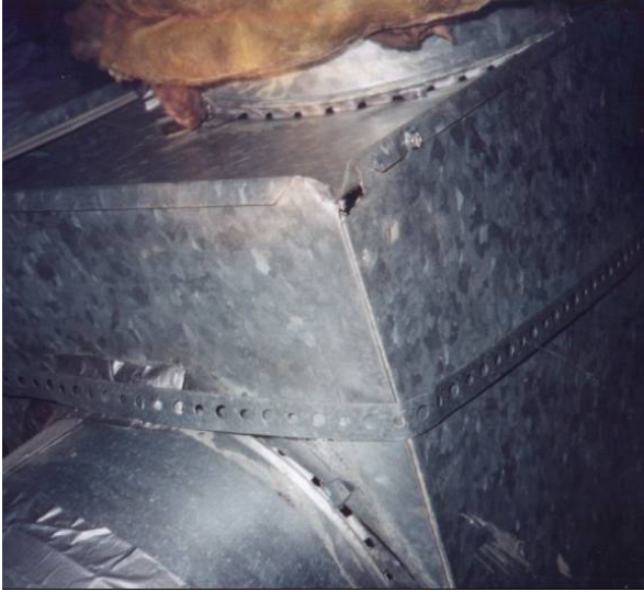
Figure 1. Field observation of a collar-to-plenum connection where the tape sealant has fallen off, and a collection of collar-to-plenum test samples from LBNL testing.
