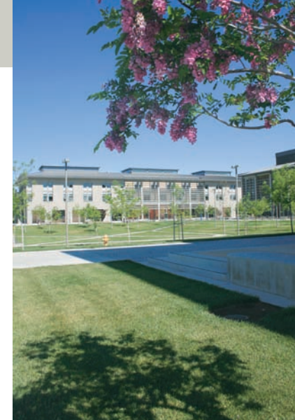
Above The UC Merced Classroom and Office Building's primary features contributing to low energy use are high performance HVAC and lighting designs and an energy management control system.
