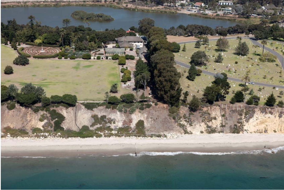
Figure 2.10: Active Cliff Erosion along the Clarke Estate and the Adjacent Cemetery
