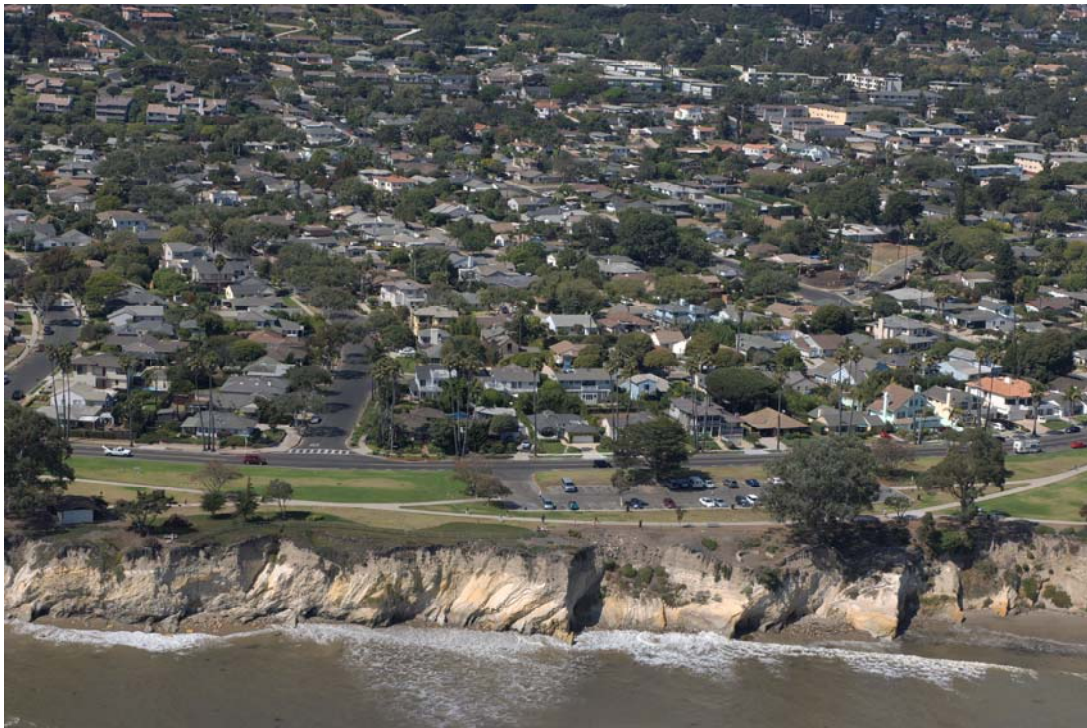
Figure 2.6: Dip Slope in the Monterey Shale along the Shoreline Park Coastline, which Produces Conditions That Are Conducive to Slope Failure
