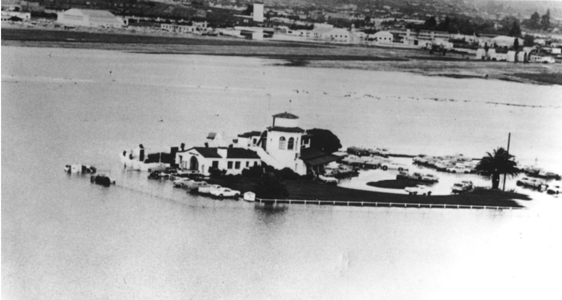
Figure 2.26: Flooding of the Airfield in 1969
