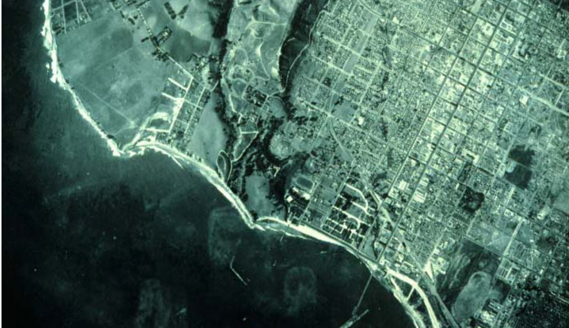
Figure 4.1: Santa Barbara Offshore Breakwater under Construction in 1928. Note the area between Leadbetter Point and Cabrillo Point and the position of the seacliff prior to sand accumulation upcoast of the breakwater.
