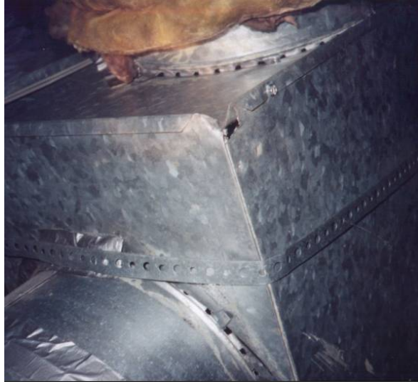
Figure 1 Example Of Collar-To-Plenum Connections On A System Where The Tape Sealant Has Fallen Off
