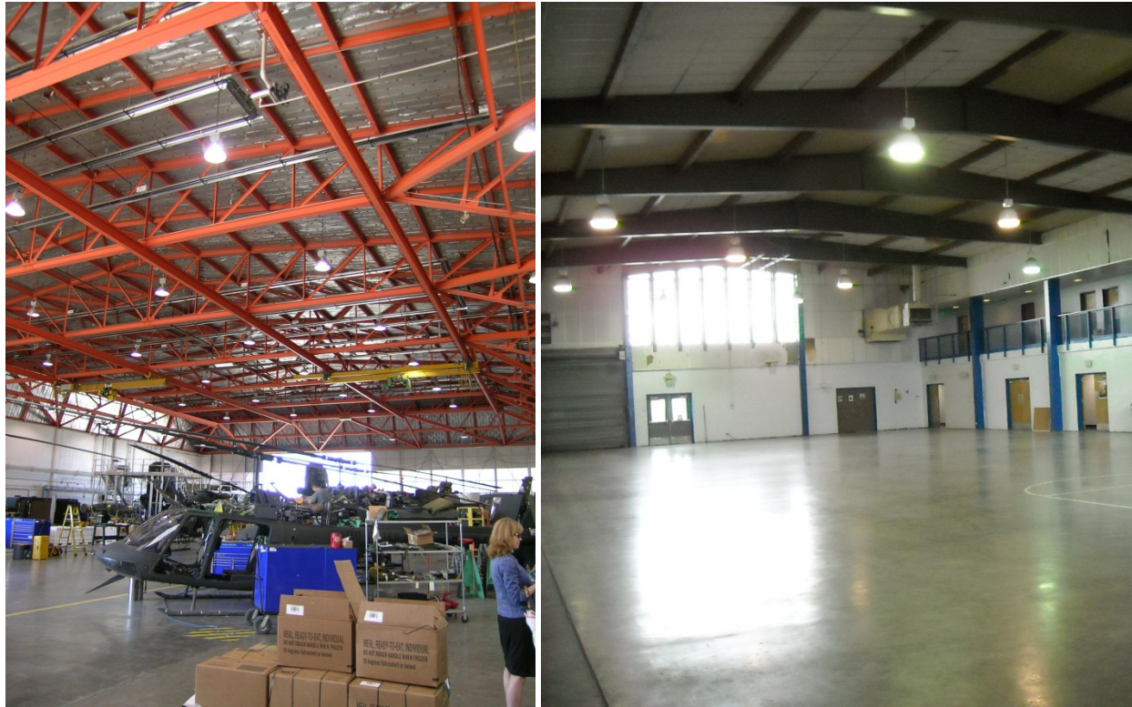
Figure 1: Incumbent high bay luminaires – main hanger (left) and work bay (right).
