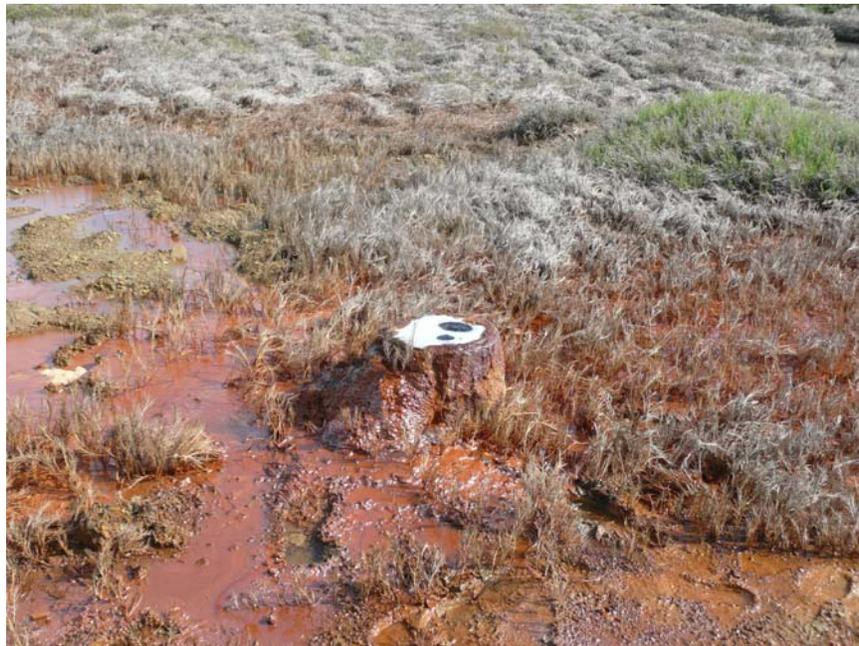
**Figure 4. Photograph of the Nurse Slough Rd. abandoned artesian well with natural gas bubbles and foam at the open well head.**
