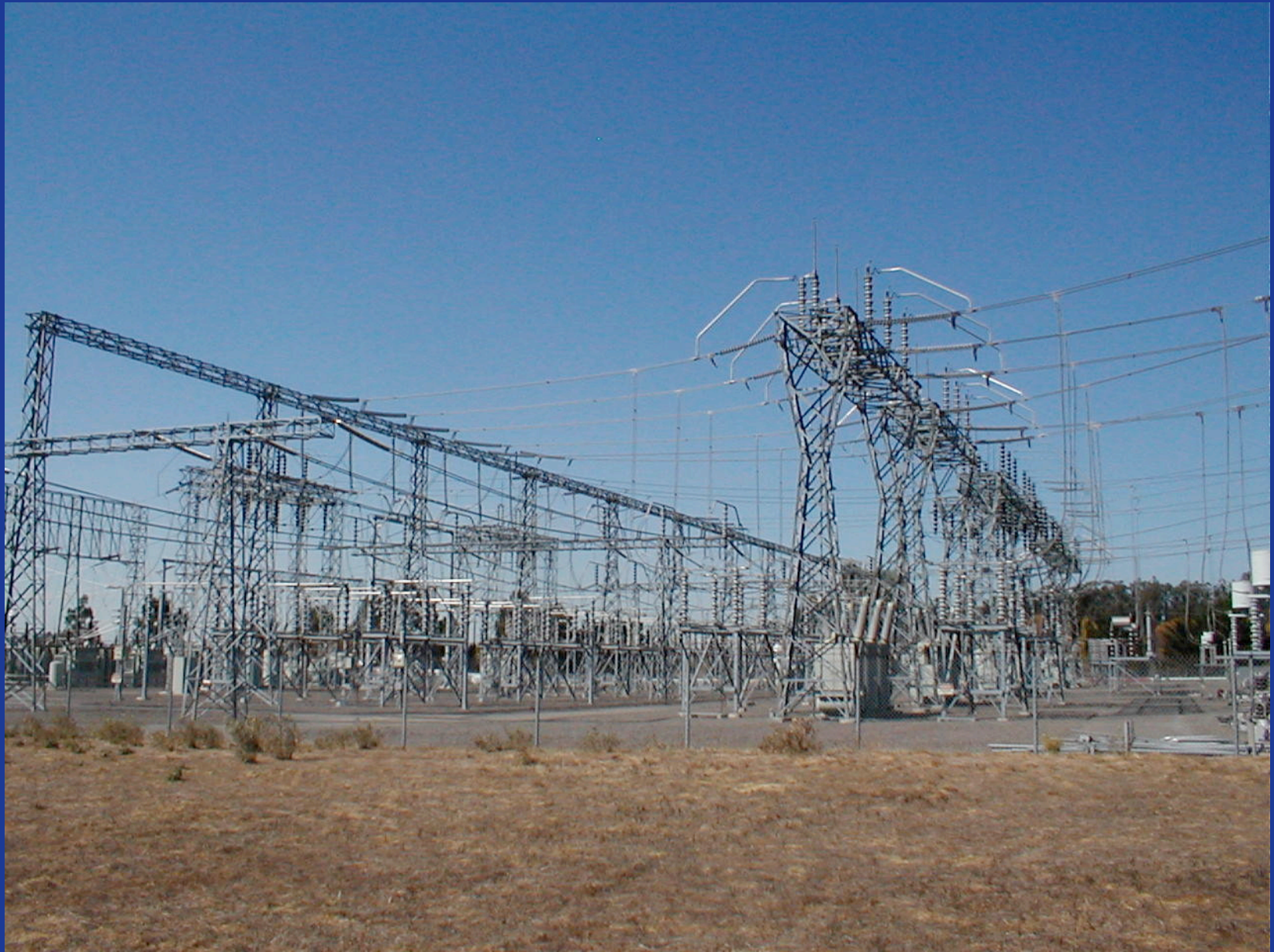
Lakeville Transmission Substation
