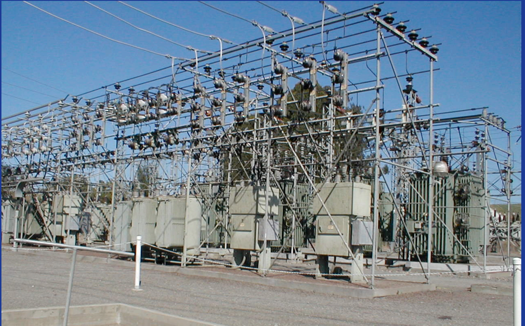
Busbars, transformers and circuit breakers at Cotati substation
