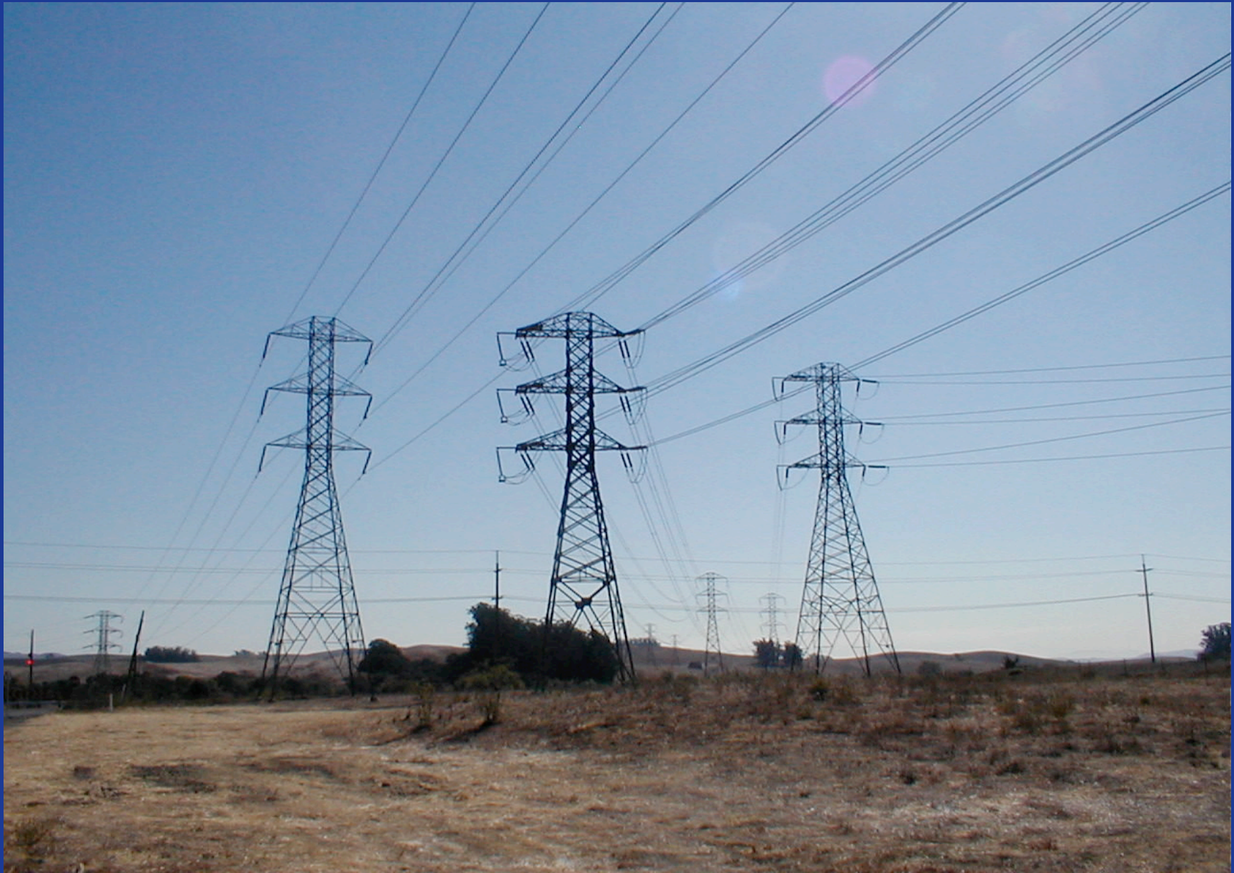
Transmission lines (230 kV)
